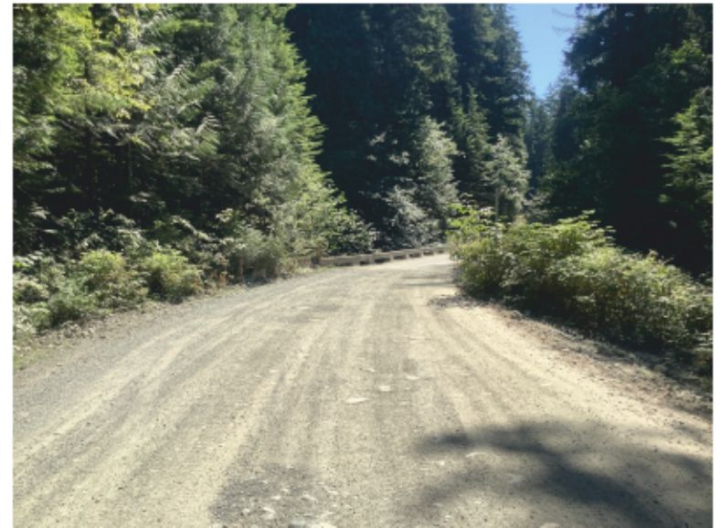
Approach from Right Bank when facing downstream
