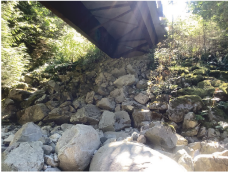
Left Bank Abutment when facing downstream
