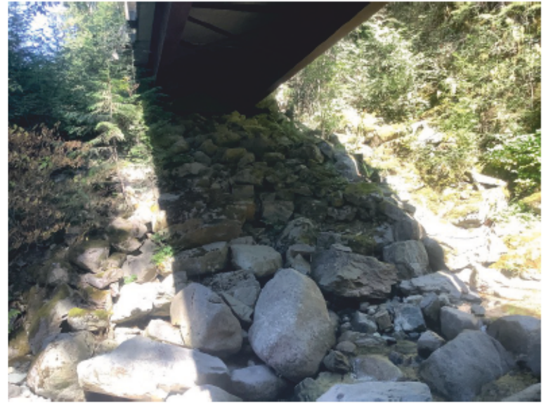
Right Bank Abutment when facing downstream
